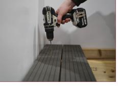
Composite decking should only be installed using correct clips and fixings. Failure to do this will affect the structure of the deck as well as warranty. Never screw directly through the boards. Steel joists >2mm must be pre drilled and specific Steel Joist Installation Kits must be used.
