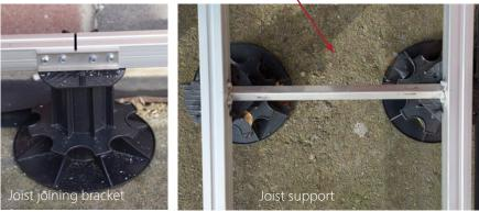
**Step 1** - Understand the spacing's required for the finished product going on top. For composite decking in residential setting using our 38mm aluminium joist, the spacing for the aluminium joist will be 400mm centres and the pedestal spacing will be 600mm.
