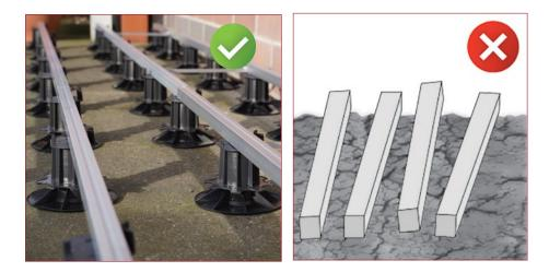
A structurally sound sub frame must be installed ensuring there is no movement prior to fixing boards to the joists. A 1.66% (1:60) fall to allow water to drain and a minimum 100mm free air space between the boards and the ground beneath to allow sufficient airflow to prevent the build up of moisture is essential.
