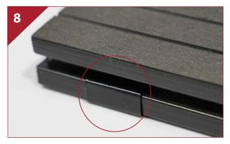
For the last row of boards use a start/end clip in line with each joist. You need to use these clips even if you putting on a fascia board. If you can not slide in the board, the boards can be fixed with screw at 45 degree angle. **Important: the screw hole must be predrilled.**
