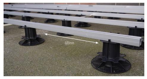
Spacing depends on joist strengths. 600mm spacing shown is for Whiteriver 38mm Aluminium Joists.
