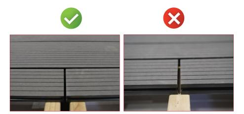
Board ends butted together must be supported by separate joists and have a min 5mm gap for expansion. Failure to do this may result in structural failure, swelling and warping. There should be a spacing gap left between the double joists to allow rainwater/debris to fall through the boards.
