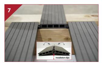
If not framed by wall or building on each side, the second last row of boards can be slid into position after you have fixed the last row and the clips for the second last row have been fixed into position.
